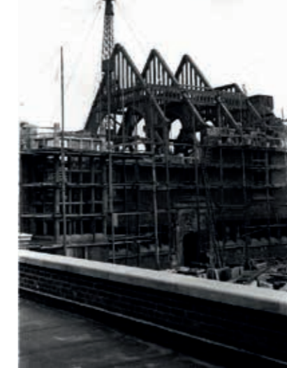
Big School under construction
